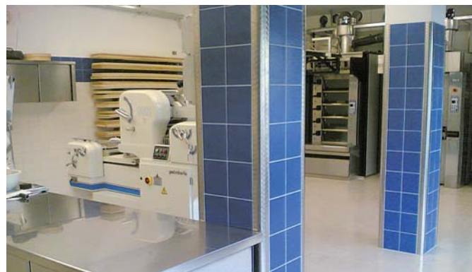
Laying example of rayed corner guards - Draw. N° 1001
